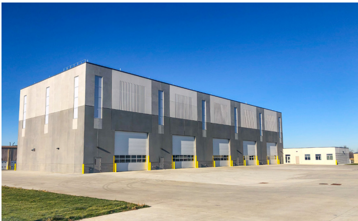
S-48 Vehicle Maintenance Instructional Building, IAARNG Camp Dodge, Johnston, Iowa
